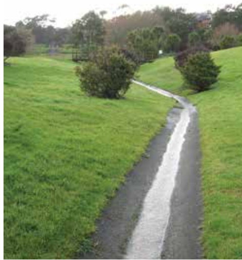
Ambitious council-led projects have turned lifeless stormwater channels...
